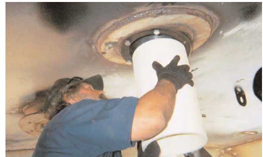
Installing SXL rudder bearing
